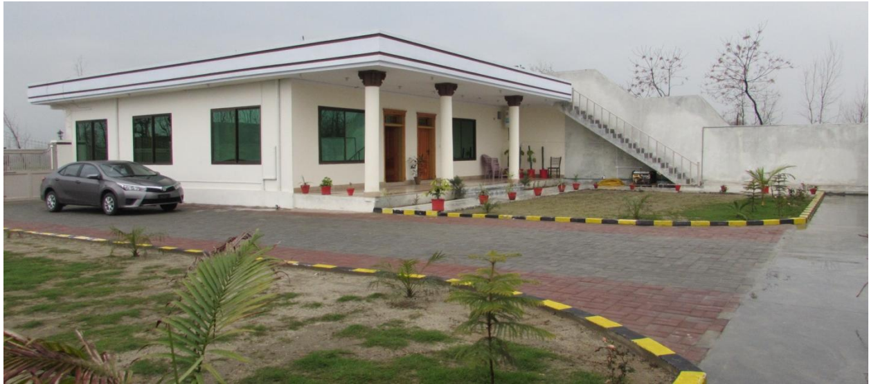
Figure 2 : Administration Block View
