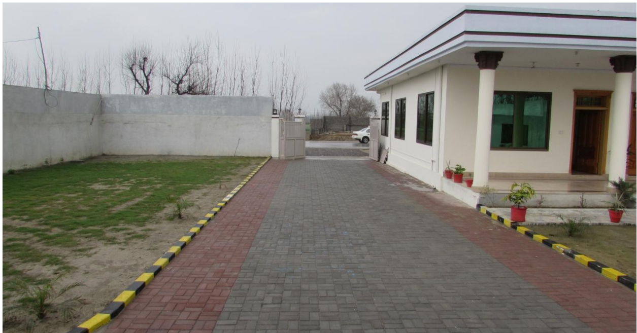
Figure 3: Main Entrance View
